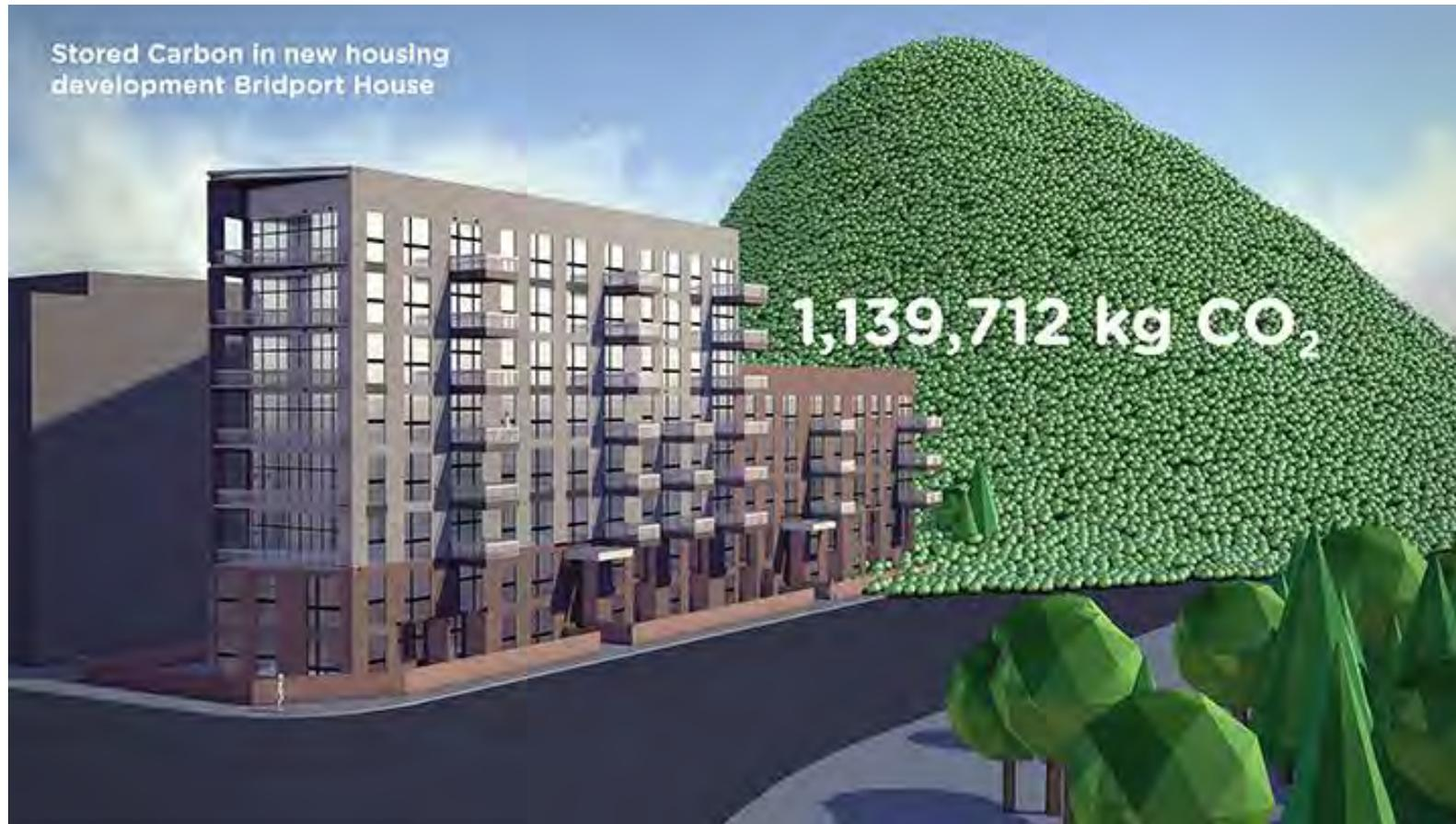
Bridport House, the UK's first multi-storey building to be constructed using only timber, is an eight-storey social housing tower in Hackney constructed from cross-laminated timber (CLT). 1,536 m<sup>3</sup> were used in construction, storing 1,139,712 kg of CO<sub>2</sub>
